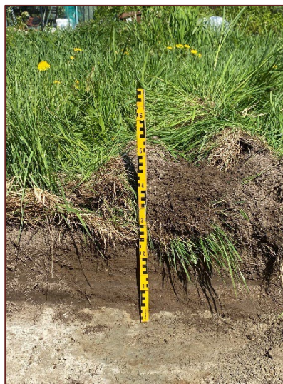
Figur 12. Ploglager i schakt 13.
